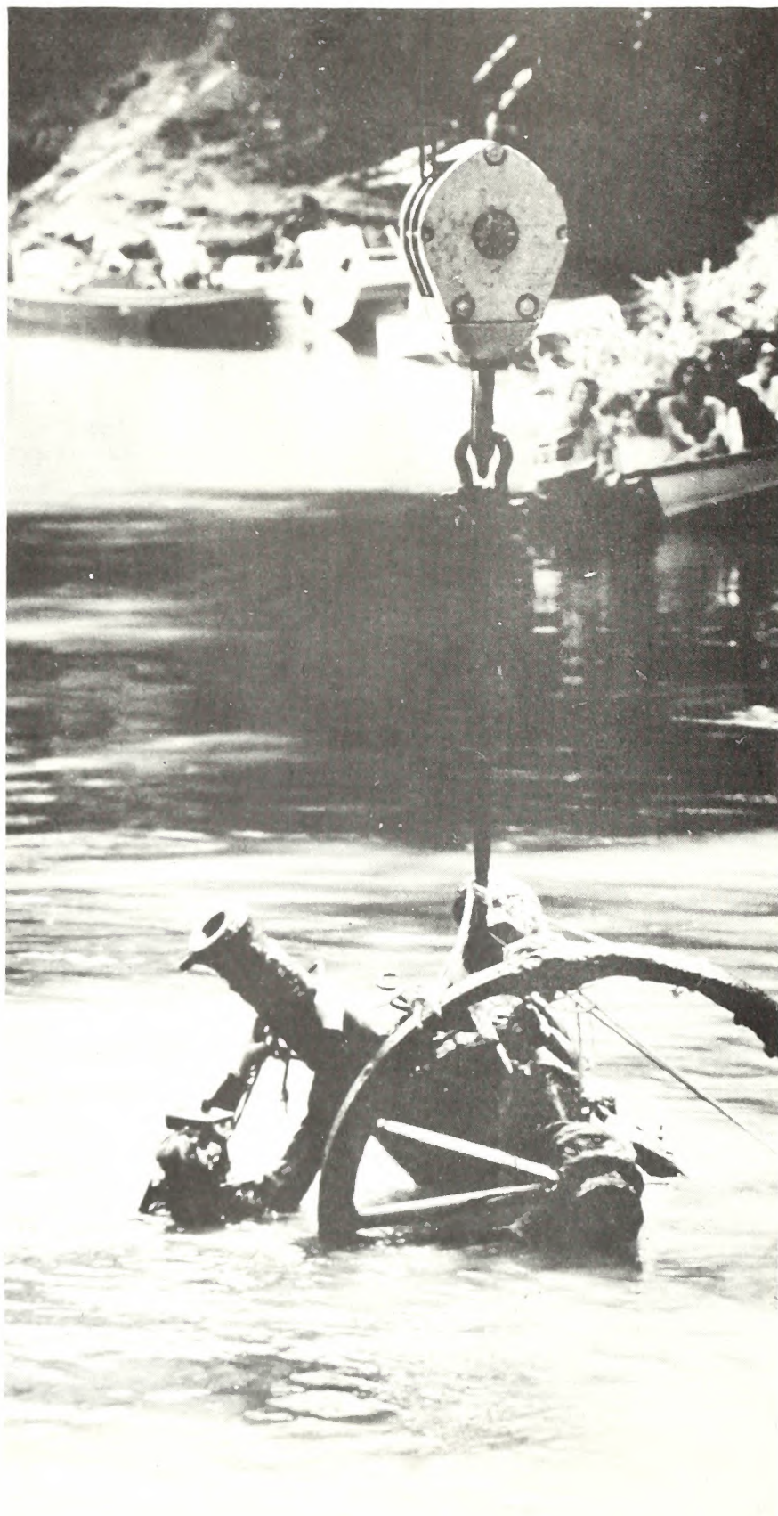
Figure 32. Diver checking lifting straps at surface
